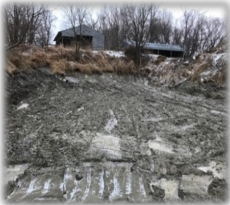
Above: Excavated pit unused for over a decade, before closure in Todd County. Prior to excavation, the inside of the pit appeared solid and grown in with grass– maybe 4 feet in depth. Surprise to all parties involved when the excavator poked through the upper crust to a depth of ten feet and mucky liquid below. The pit was in close proximity to a river and playing children.
